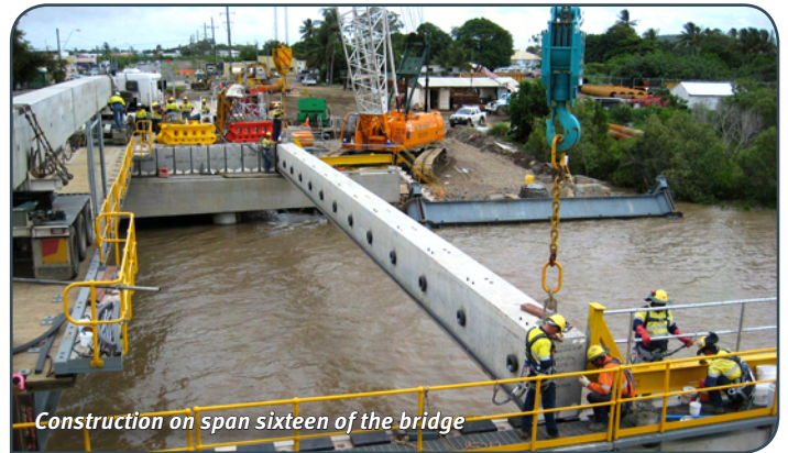
Placing deck units on the Forgan Bridge
